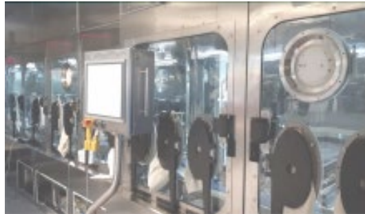
Injectable line in Barcelona plant
